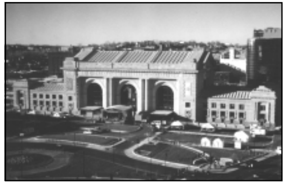
ABOVE—Union Station soon after Science City opened in 1999. Amtrak’s former home (1985-2002) was behind and below the tall building at right, whose construction blocked the old track area.
